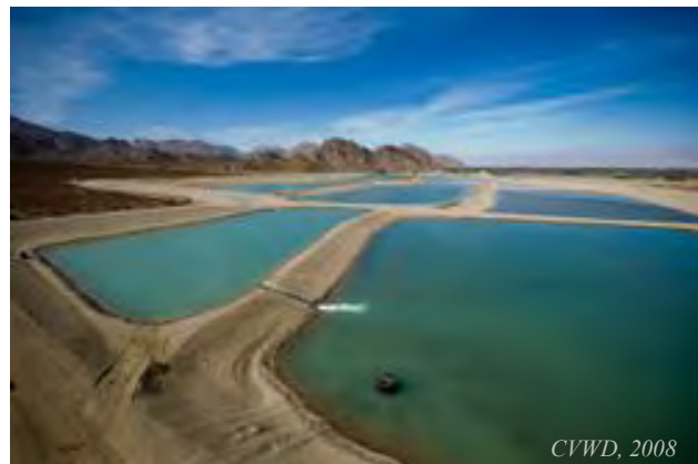
Groundwater recharge areas at the Thomas E. Levy Groundwater Replenishment Facility
