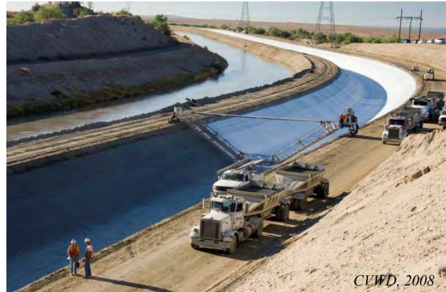
Coachella Canal lining project
